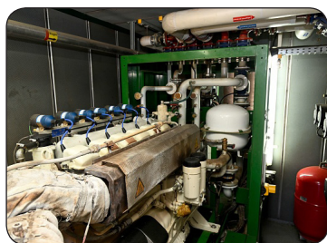
A biogas reciprocating engine generator installed on a farm
