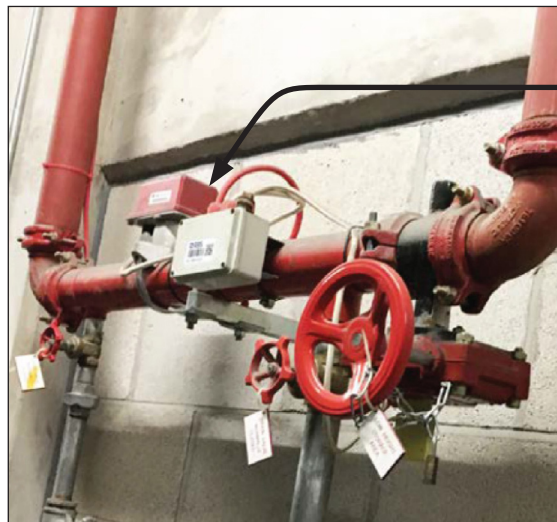
Flow switches to be checked quarterly
