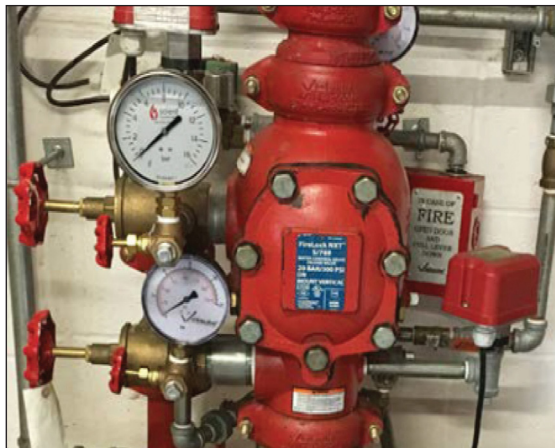
Typical 'Pre-Action' Control Valve Set
