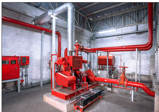
Photograph shows horizontal split case diesel fire-pump
