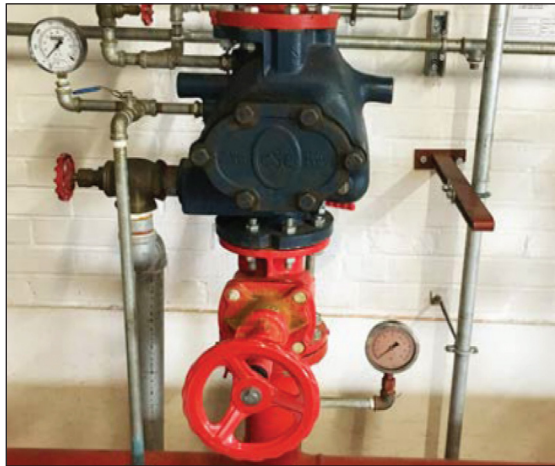
Typical 'Dry' Control Valve Set
