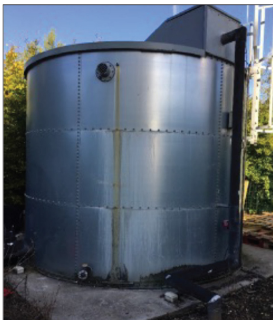
Photograph shows a typical cylindrical '10-year' sprinkler tank
