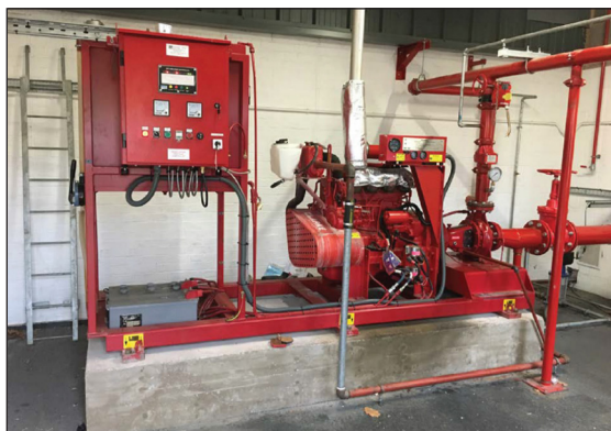
Photograph shows typical end-suction diesel fire-pump
