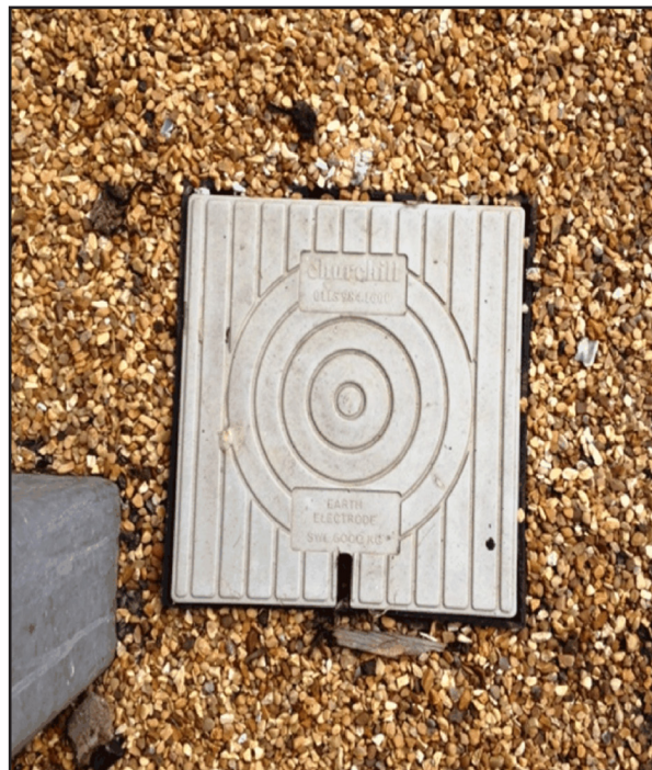
Figures 3 and 4: Each down conductor should be provided with an earth terminal (5.3.2)
