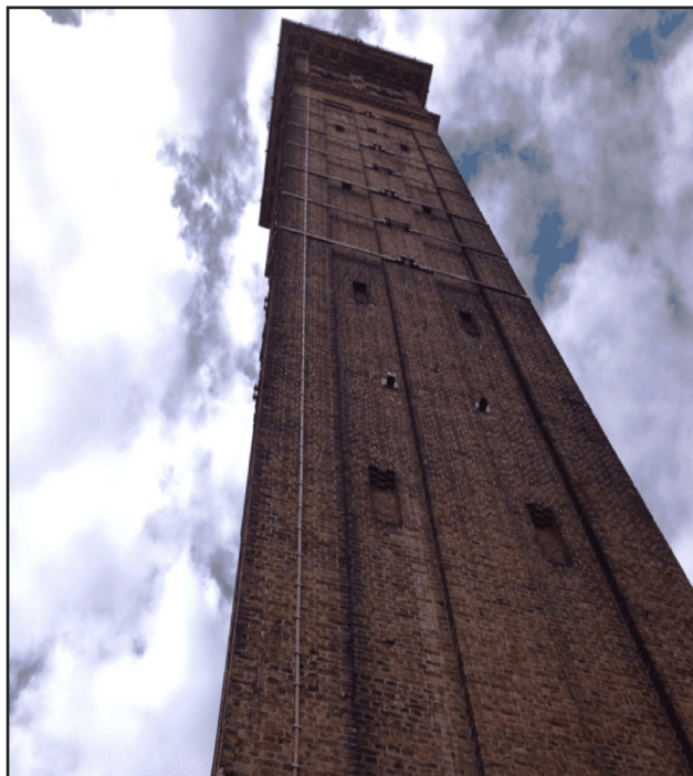
Figures 3 and 4: Each down conductor should be provided with an earth terminal (5.3.2)
