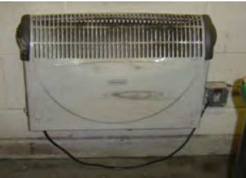
Figure 6: If a loose lead on a fixed heater is accessible the heater should be included on the in-service testing programme (5.5.13)
