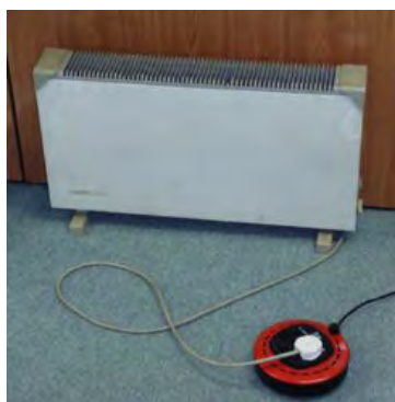
Figure 5: The use of extension leads to provide power to electric heaters should be avoided (5.5.7)
