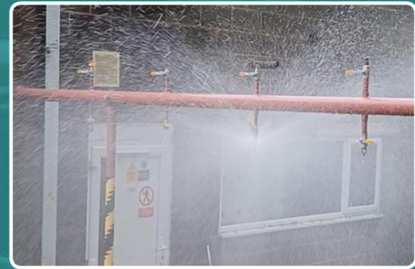
**Deluge:** uses open sprinkler heads and delivers water to all simultaneously upon activation (not considered in the LPC Sprinkler Rules).
