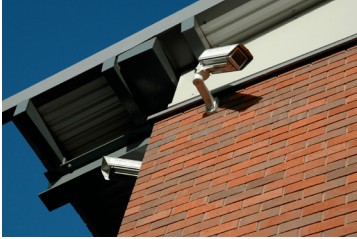
Figure 21: Camera viewing an area with public access (courtesy BSIA)
