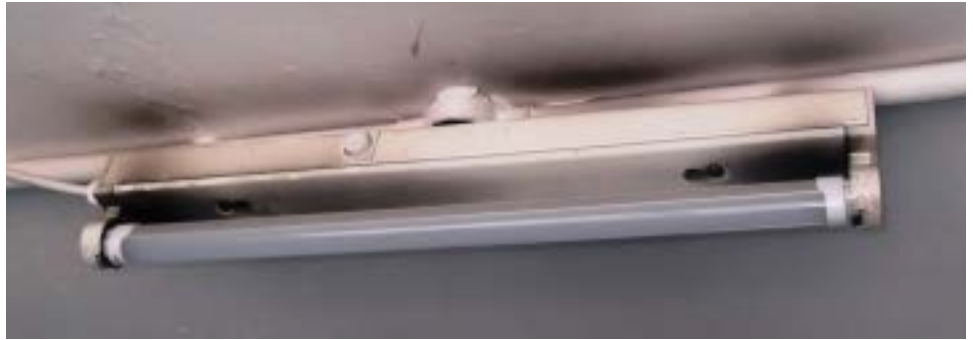
Figure 6: Overheating fluorescent light
