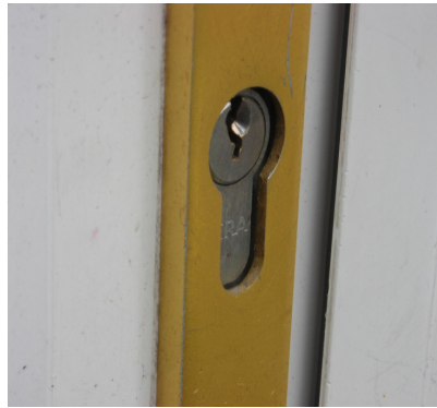
This cylinder is too short, leaving the door furniture more vulnerable to being gripped and broken away
