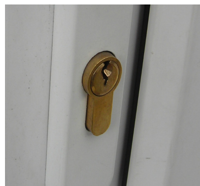
This cylinder protrudes slightly, so may be vulnerable to a snapping attack
