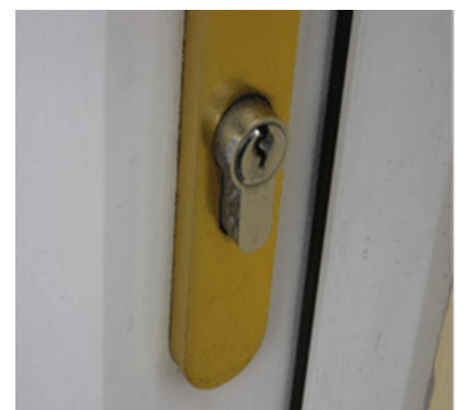
This cylinder protrudes several millimetres and is very vulnerable to a snapping attack
